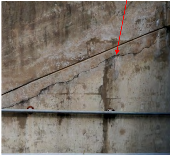
Cracks at south ramp wall do not appear to have been repaired via epoxy injection
