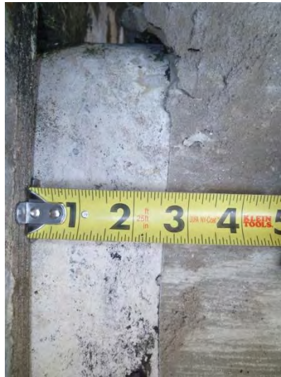
Vertical and horizontal separation of isolated deck and supporting beam at north intermediate expansion joint (East Stadium, View from Below Deck)
