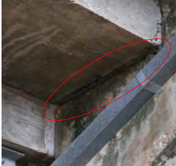
Vertical and horizontal separation of isolated deck and supporting beam at north intermediate expansion joint (East Stadium, View from Below Deck)
