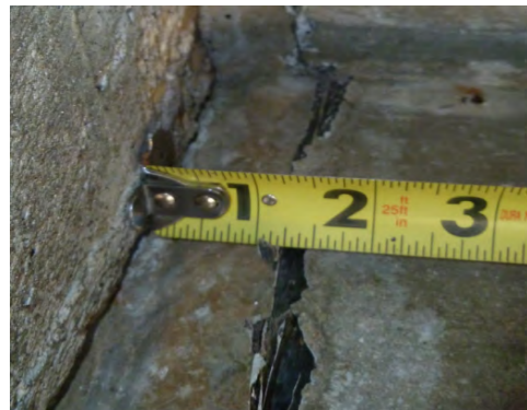
Horizontal separation of supporting beam and isolated deck
