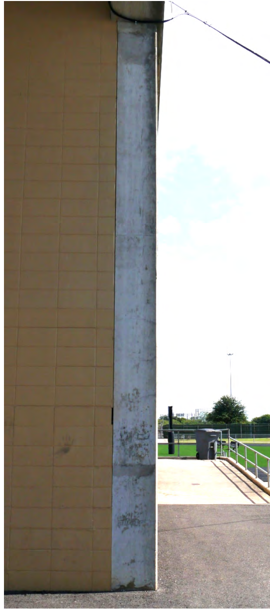
Lateral deflection at top of column – top portion of column has separated from CMU wall
