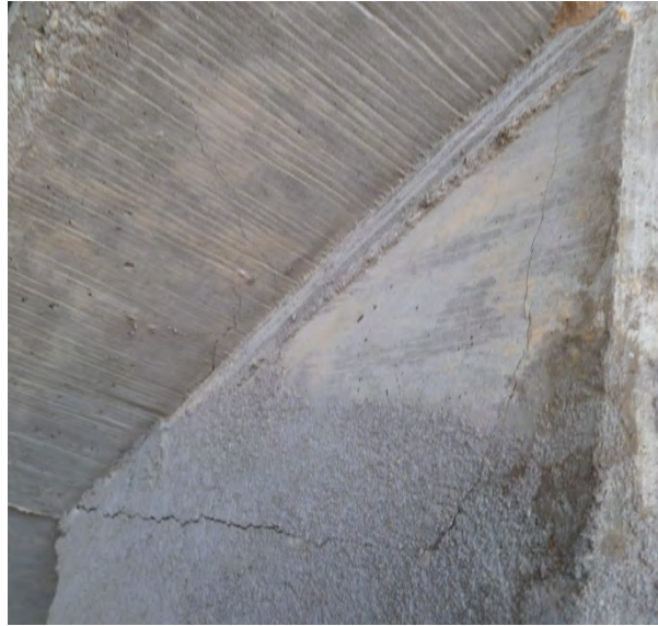
Previously repaired cracks at top of column have re-opened and new cracks have developed
