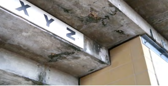
Significant cracking in deck and joists; Water stains due to water infiltration thru deck cracks
