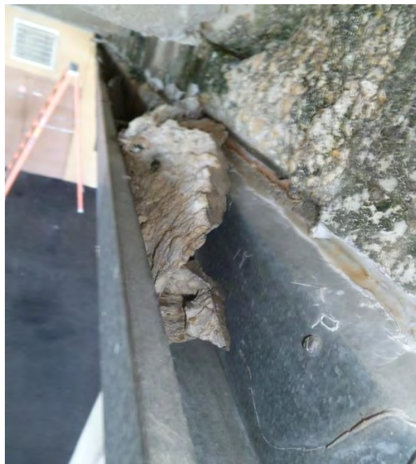
Spalled beam concrete caught in the gutter
