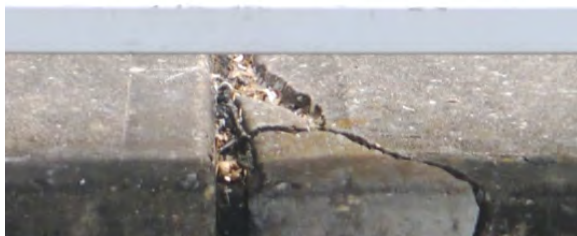
New concrete damage at expansion joint (since 2006 repair work)
