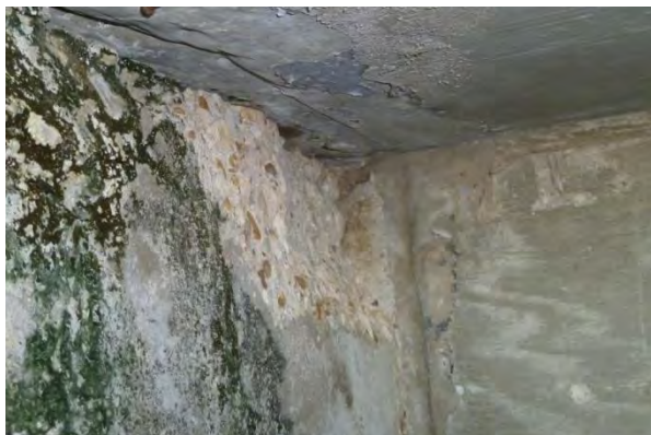
Vertical gap between supporting beam and isolated deck
