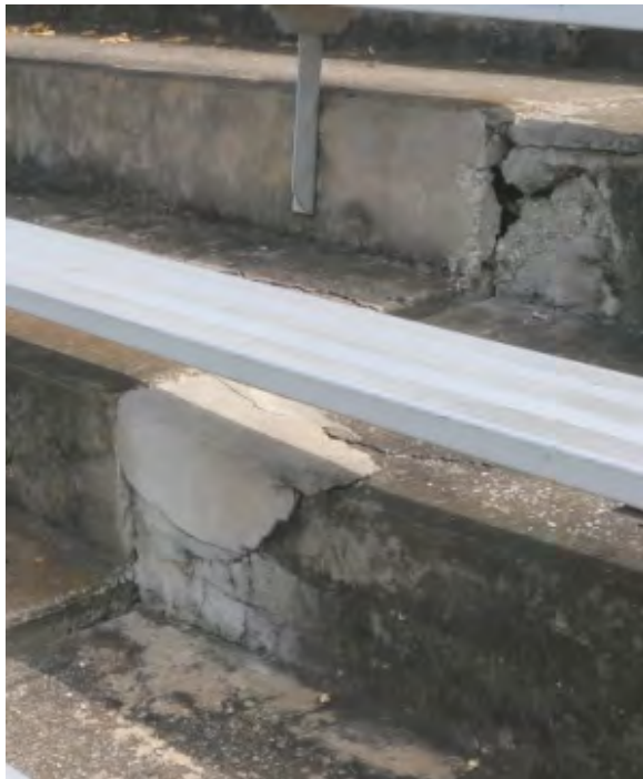
Horizontal & vertical separation at south expansion joint; New damage at previously repaired concrete (East Stadium, View from Top of Deck)
