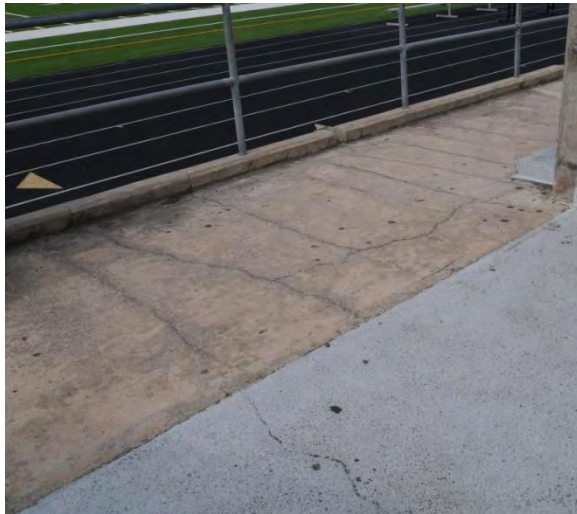
Prevalent cracks on top of deck allow water to infiltrate the concrete & exasperate progression of damage
