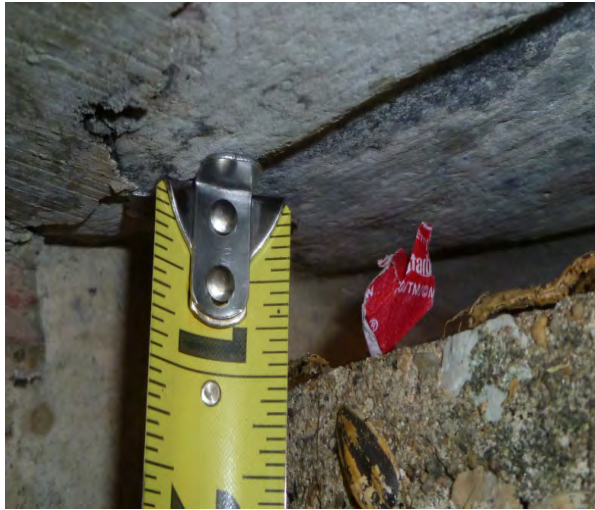
Vertical gap between supporting beam and isolated deck
