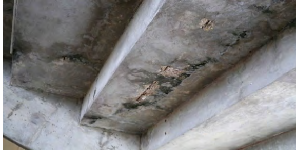
Spalling with exposed/corroded reinforcing at underside of deck; Water stains due to water infiltration thru deck cracks
