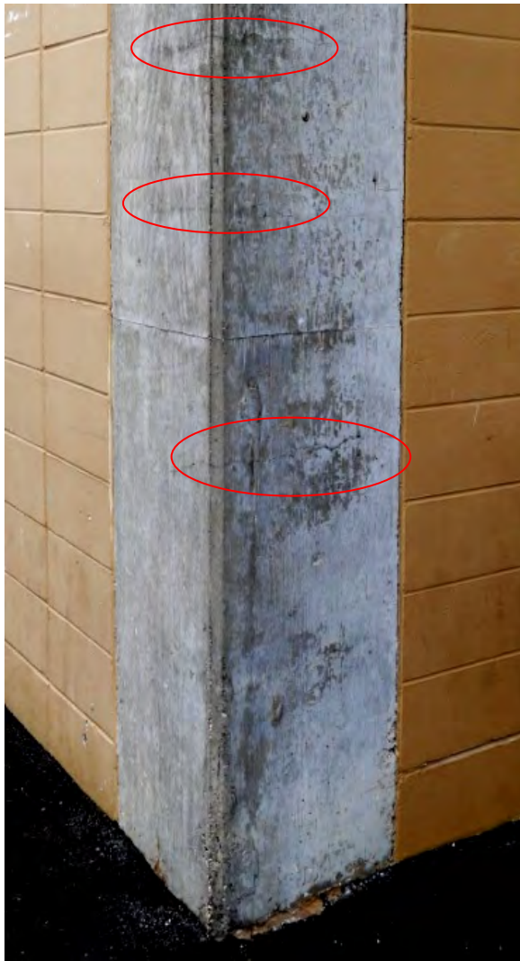
Flexural Cracking Near Bottom of Column
