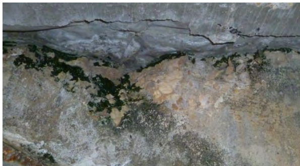
Concrete at the top corner of the supporting beam is spalling (below isolated deck)
