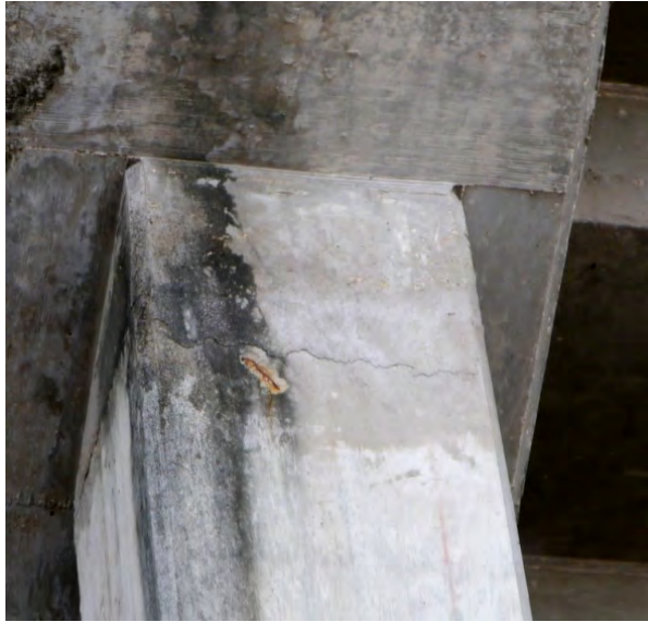
Previously repaired cracks at top of column have re-opened
