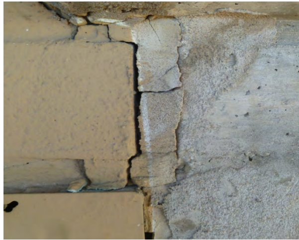
Edge column has separated from CMU wall
