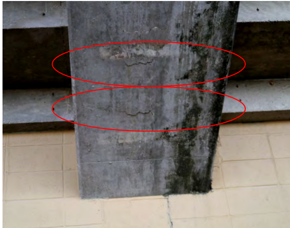
Cracked beam soffit
