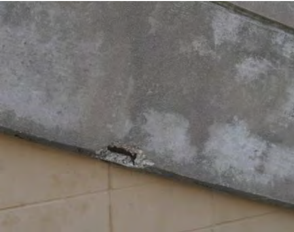
Exposed/corroded beam reinforcing
