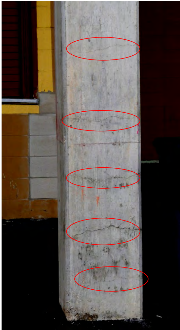
Flexural Cracking Near Bottom of Column
