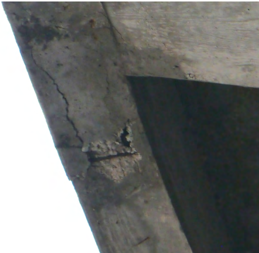
Failing concrete repair patch on beam soffit; Exposed/corroded beam reinforcement
