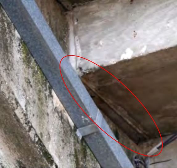
Vertical and horizontal separation of isolated deck and supporting beam at south intermediate expansion joint (East Stadium, View from Below Deck)
