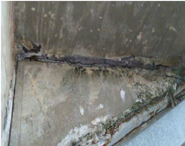
Horizontal separation of the supporting beam and isolated deck
