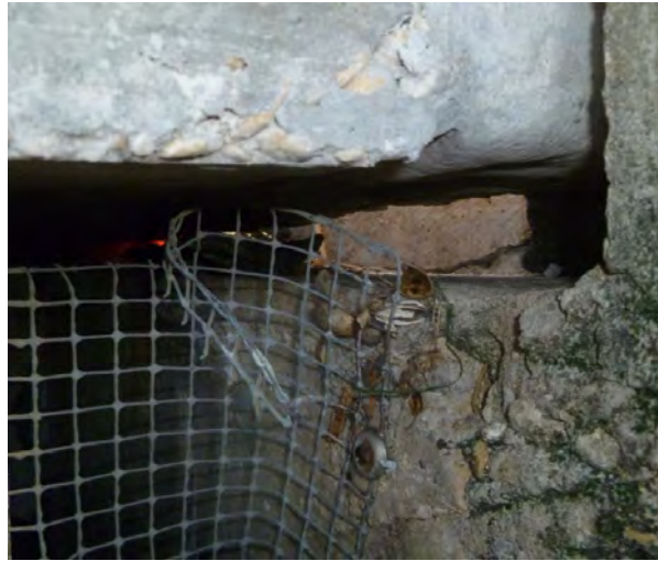
Daylight visible between supporting beam and isolated deck
